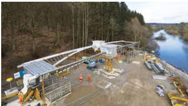
Site assembly. Image courtesy of WEC Group.
