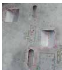
Corroded areas cut and prepared ready for repair welding.
