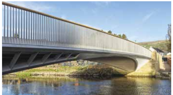
The bridge – installed. Image courtesy of WEC Group.
