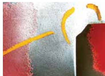
Figure 2: A weld, stripped of paint for inspection purposes.
